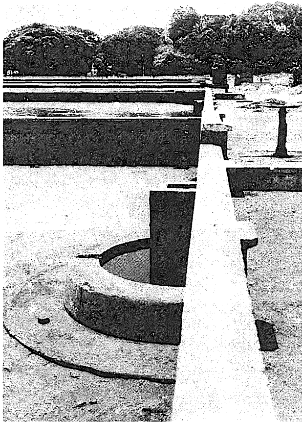
FIG. 24. CONCRETE APRONS TO PREVENT SCOUR AT INLET TO SLOW SAND FILTER MADRAS WATERWORKS, INDIA
